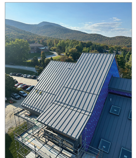
Courtesy Mountain Green Condo Association New roofing is planned to seal the envelope of all three condo buildings.
