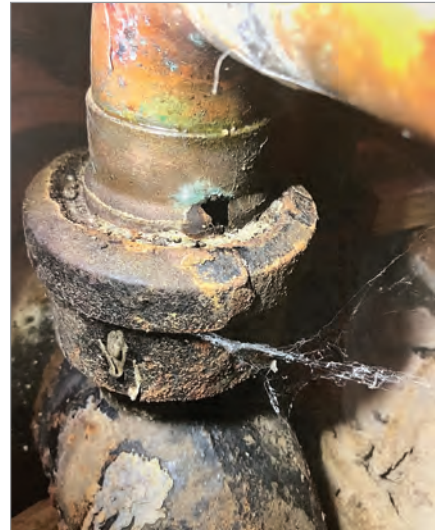
District Buildings and Grounds Manager Joe Rigoli shows areas of erosion, corrosion, and moisture damage, along with other factors, that have led to risk of complete system failures during a recent walk-through tour of The Woodstock Union Middle-High School building. The next tour will be offered Tuesday, Nov. 28 at 6:30 p.m.
