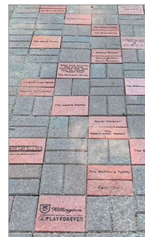
Courtesy Jim Haff Nearly 80 donors received a monogrammed brick embedded in the walkway to the new playground.
