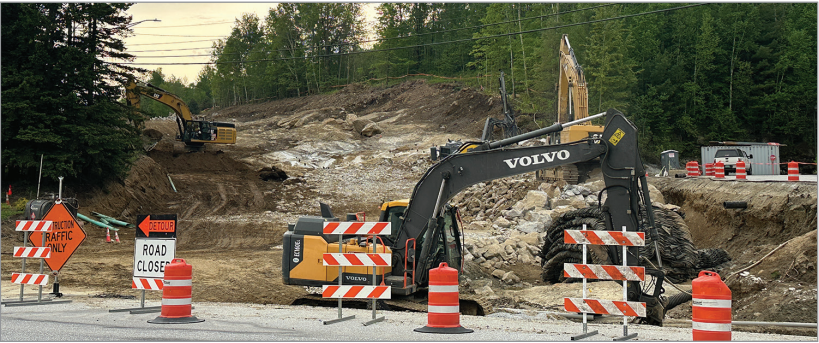
By Polly Mikula Reconstruction of Killington Road continues at its intersection with Route 4. Blasting occurs once a day between 11 a.m. and 1 p.m. in order to level the entrance.
