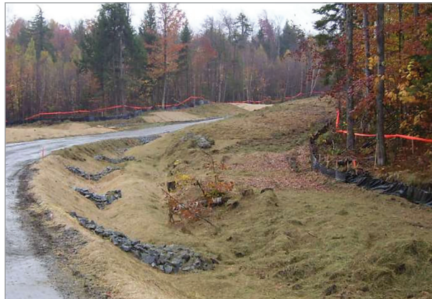
Top: Barrier tape marks the limits of the construction site. Bottom left: Stone or rock check dams slow erosion in drainage channels. Bottom right: Filter socks (a manufactured tube filled with shredded material) slow stormwater runoff on long open slopes.
